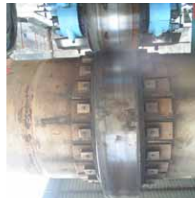
Repair of kiln tyre/ bearings
