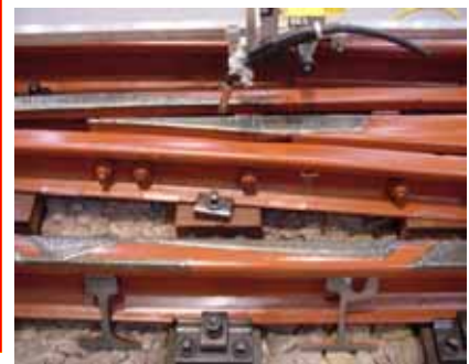
Repair rails/ crossings/ends
