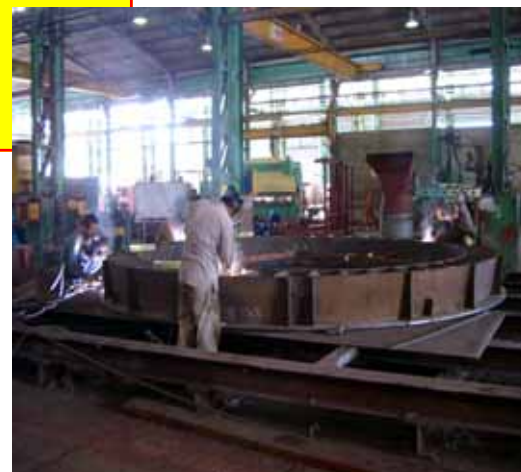
Containers and tanks
